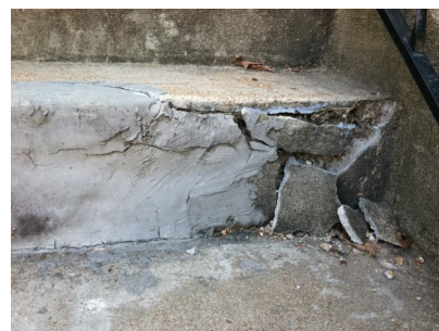
Broken or crumbling stairs need to be repaired to preserve the health and safety of residents and visitors. Photo credit: oldhouseweb.com
